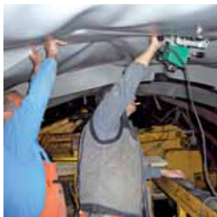
Comet operating in the tunnel ...
