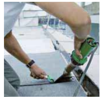
For welding of bitumen sheets, use the powerful ELECTRON with wide slot nozzle.
