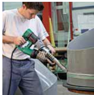
The FUSION 3C in operation during container construction.
