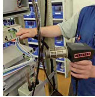
Simple heating up fibre optic loose tube cables for further processing.
