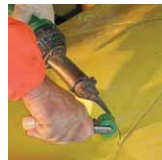
The hand roller is an essential accessory for tunnel applications.
