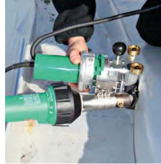
The TRIAC DRIVE PID even allows horizontal welding.
