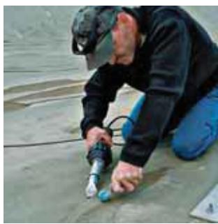
Welding of the connectors with TRIAC PID and push-fit wide slot nozzle.
