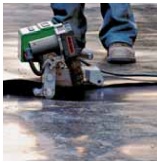
TWINNY T with combiwedge, welding a HD-PE sealing sheeting.
