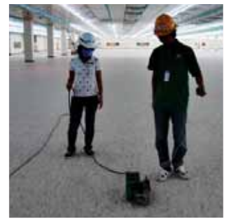
Immaculate weld seams with the UNIFLOOR E (Vietnam).
