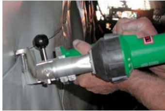
TRIAC DRIVE PID welding a horizontal seam in tunnel construction.
