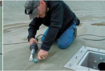
Welding connections using TRIAC PID with push-fit wide slot nozzle.
