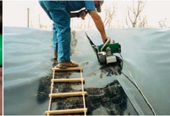
ASTRO achieves perfect welding seams even at the highest speed of 5 m/min.
