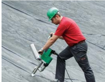
Without welding rod: The WELDPLAST G6 is with its granulate funnel an independent partner.
