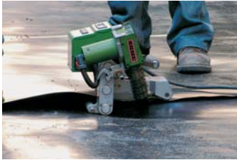
TWINNY T with combi-wedge used to weld a HD-PE liner.
