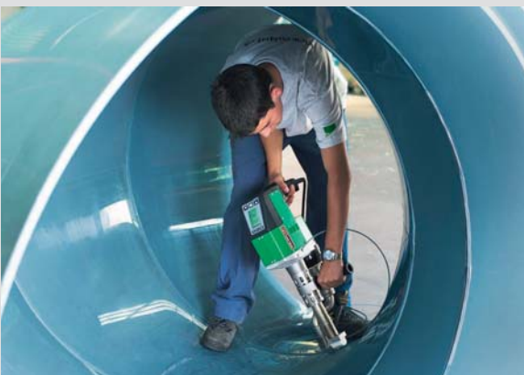
Pipeline manufacture with WELDPLAST EC4
