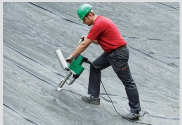
Landfill site construction with WELDPLAST G6 (with gran late funnel)
