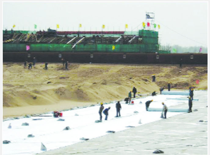
Daily the surface area of two football fields are sealed with HD-PE Geomembrane.
