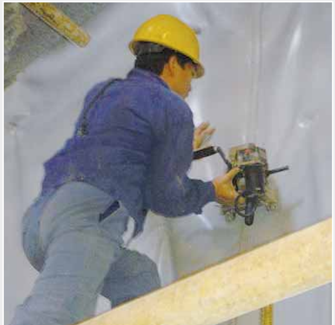
The light, handy TWINNY S brings the weld seam down almost by itself...
