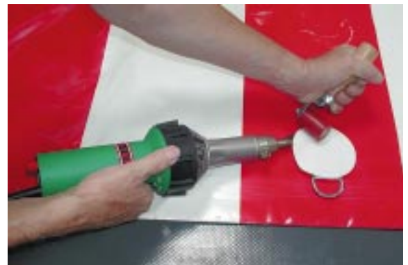
Welding tie downs with Triac S.
