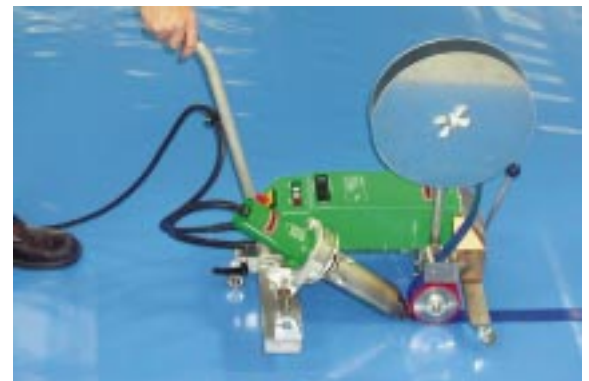
A 40 mm reinforcement tape is welded onto a PVC cover.
