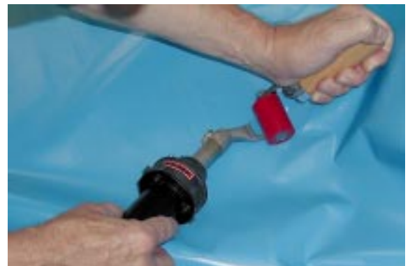
Repairing a pool cover with HOT-JET S.
