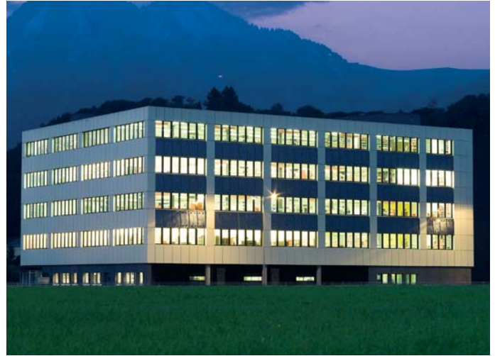
The company building in Sarnen, Switzerland
