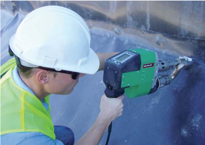
The WELDPLAST S4 whilst joining the plastic sealing tracks to the shore boarding.
