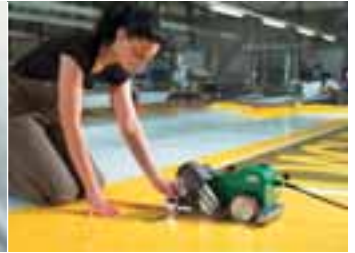
Overlap welding of a billboard with UNIPLAN E.
