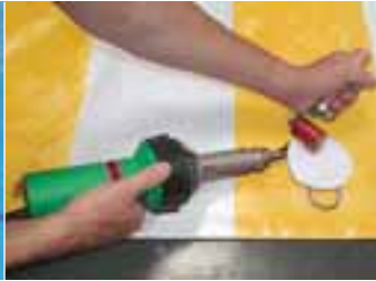
Welding tie downs with TRIAC S.
