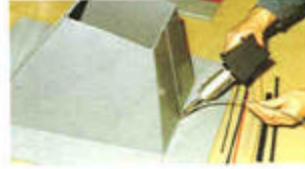
Repair & fabrication of ventilation duct work.
