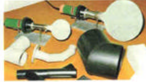
Pipe butt welding with welding mirrors.
