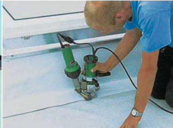
TRIAC DRIVE PID used for welding plastic roofing membranes in a light dome.
