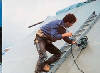
X84 used to weld an under-roof liner on a high-pitched roof. Weighing only 6.1 kg, the X84 copes with any incline at constant speed.
